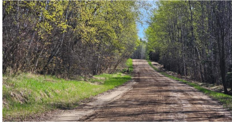
P26 TR592A – looking east
