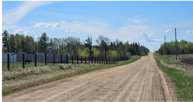
P19 RR240 – looking south
