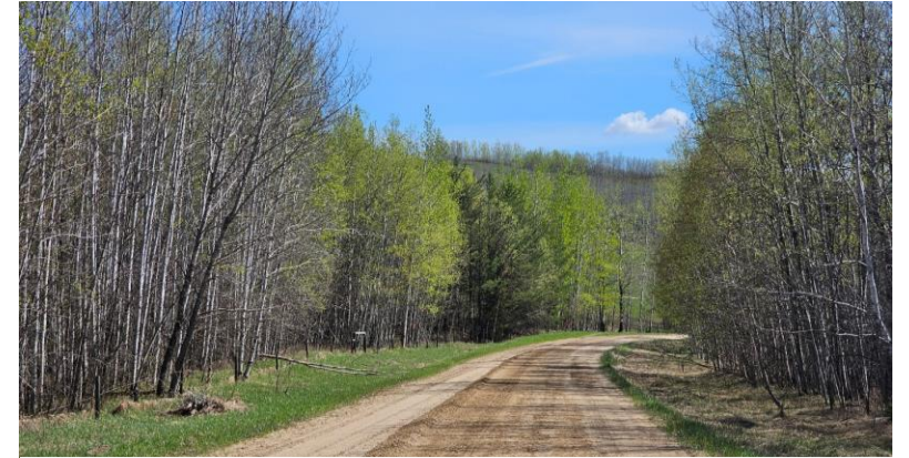
P25 TR592A – looking east
