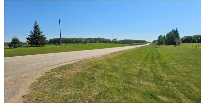
P18 RR240 / Hwy 18 – looking east
