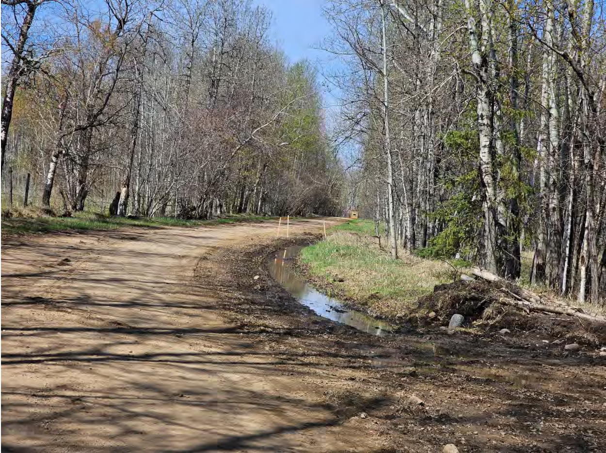
Photo P28 – Township Road 592A Looking west along Township Road 592A
