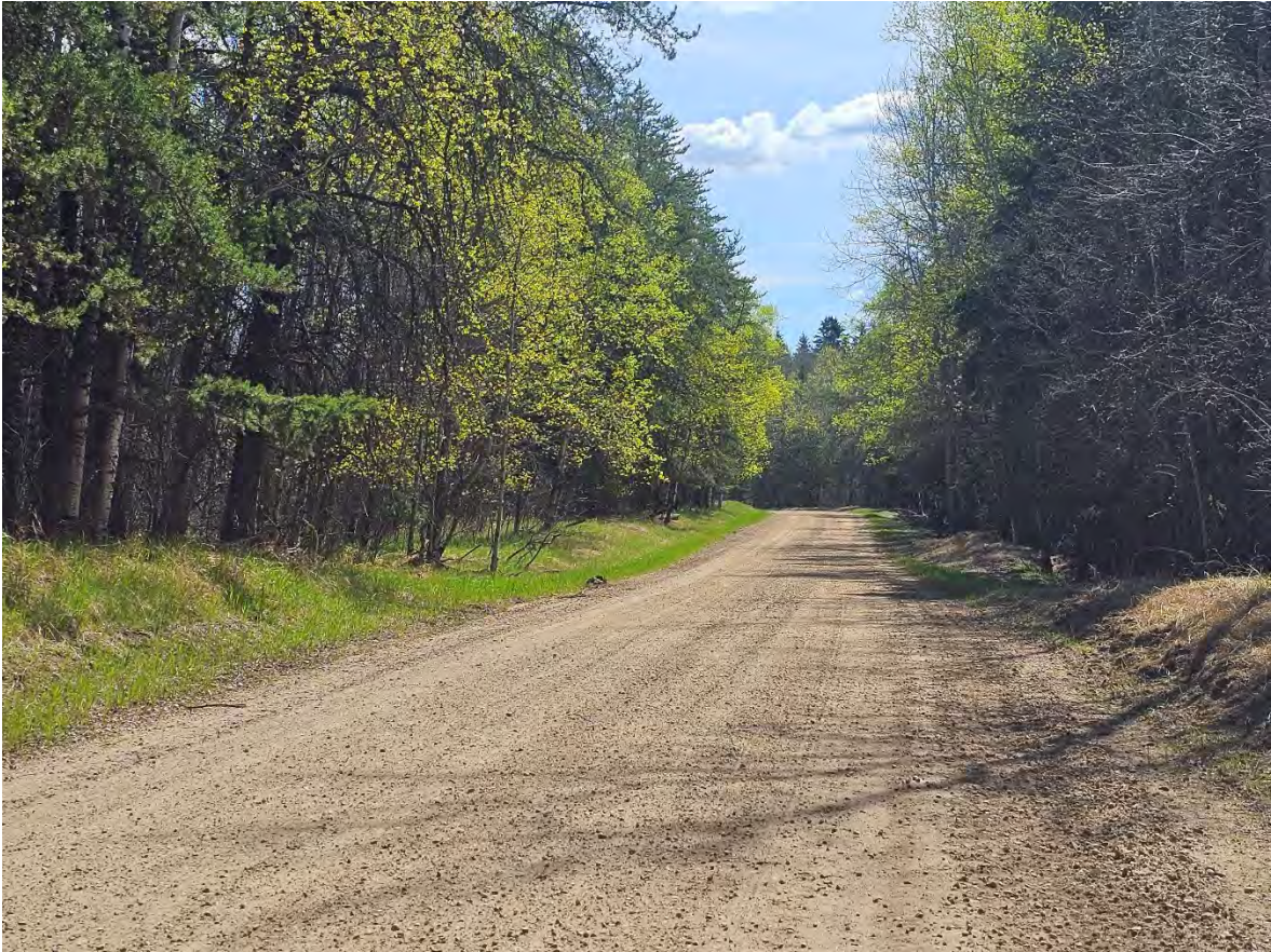
Photo P27 – Township Road 592A Looking east along Township Road 592A approaching the eastern portion of the Option 5 corridor
