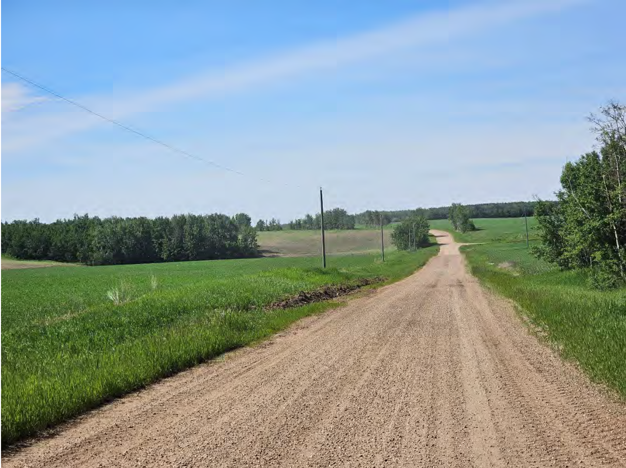
Looking south along RR240A
